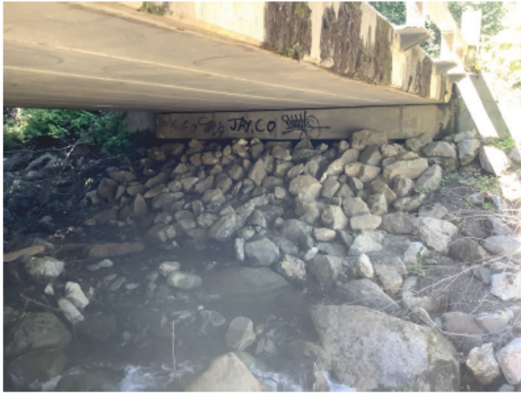
Left Bank Abutment when facing downstream
