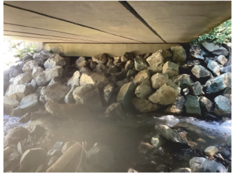
Right Bank Abutment when facing downstream
