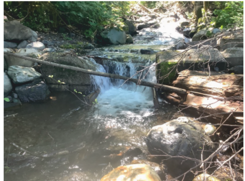
Old weir structure upstream
