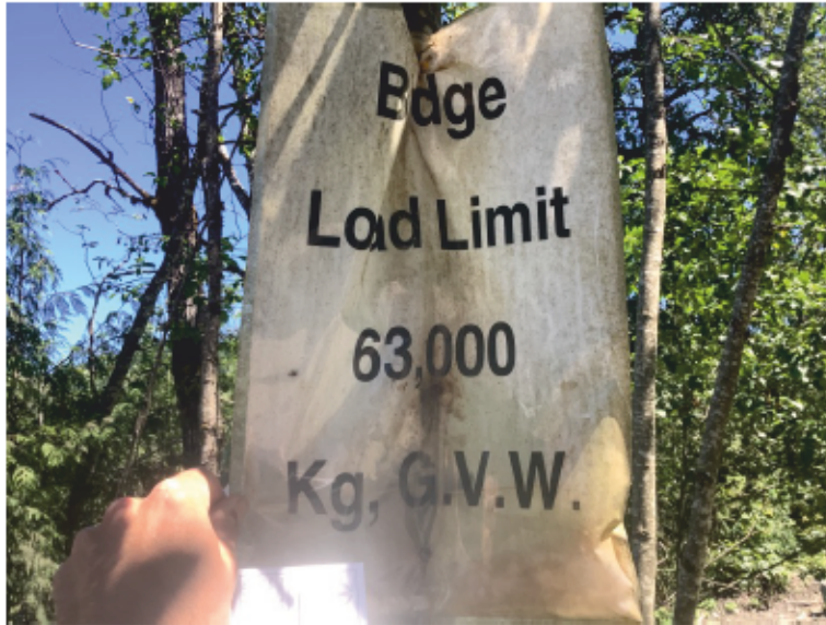
Load Rating Sign
