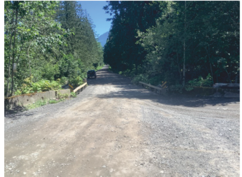
Approach from Left Bank when facing downstream
